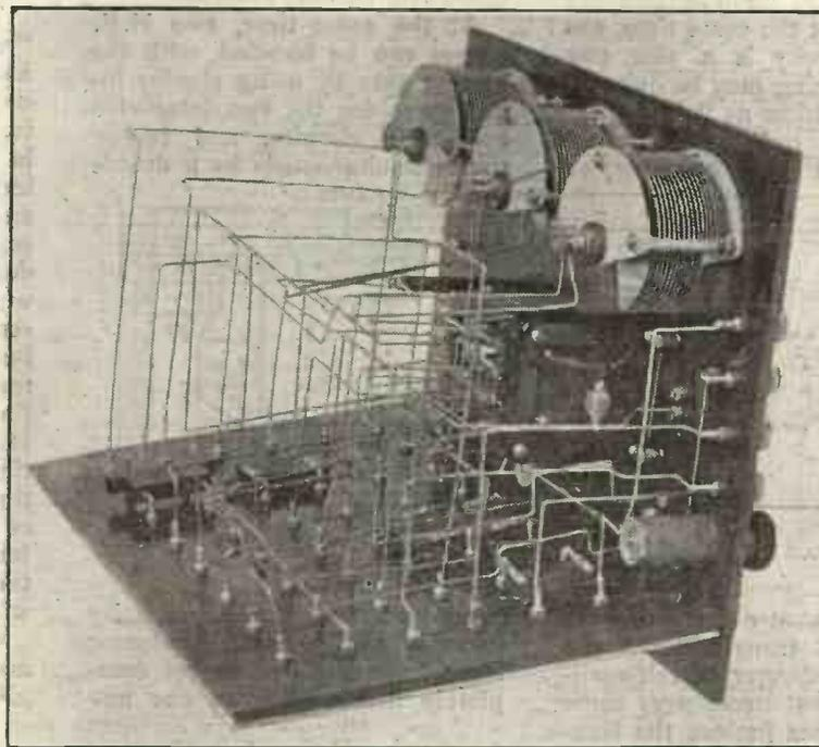
Back view of the Omni-Circuit Receiver, showing components and wiring.
