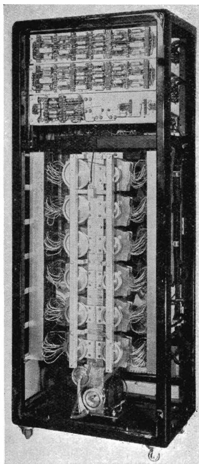
Fig. 6. Rear view of apparatus rack showing two rows of six belt-driven generators
