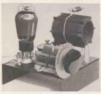
This is the original experimental chassis on which we tested the AC4| PEN. It is not essential to use such a large diameter coil, but it has one advantage, a tap-ping point can be made during the experimental stages.
