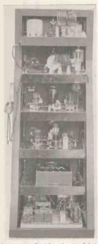
One chassis is allowed for each section of the transmitter. In this way modifications and tests can very easily be made.
