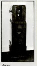
Baird's 30-line mirror drum television receiver built in 1932 by Bush.
