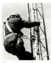
The IBA's Safety Officer, fastened to a transmitting mast by means of a special harness, tests safety procedures adopted by maintenance staff.
