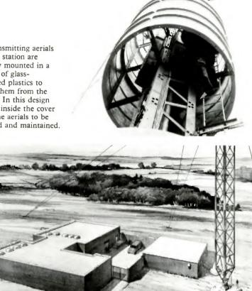
An artist's impression of a building design for a high-power television transmitting station. Once the equipment has been installed such a station will operate automatically under the supervision of a control room many miles away.
