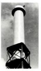
A 3ft diameter cylinder containing UHF transmitting aerials mounted in a special cradle to allow tests to be carried out near the ground. Later the complete unit will be taken to the transmitting station and lifted and fixed many hundreds of feet above ground. (*EMI*)
