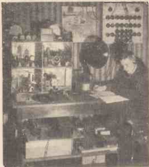
This is the transmitting gear at the Dutch station PAOHJ, which is often heard in the 80-metre band. The lead-in wires go to a Zepp aerial. Underneath you can see the modulator power pack. The second operator is at work!
