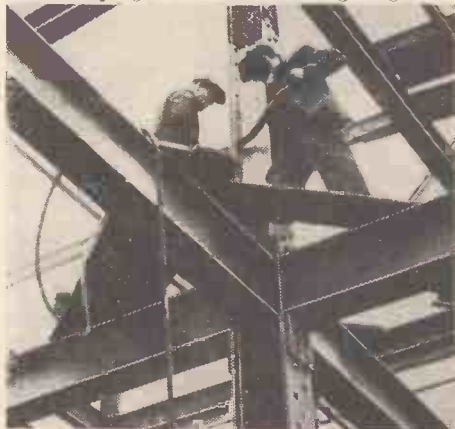
Radio marches on! Two striking views of the new Cossor factory now going up at Highbury. The height will be 75 ft. for the five storeys, for which 500 tons of British steel are needed. 60,000 sq. ft. of floor space will be available for over 1,000 workers.
