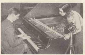
Making a record of the Neo-Bechstein piano, which makes use of microphones and amplifiers to reproduce the sounds for the strings
