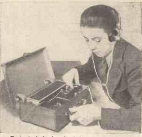
Tuning in the local station during an early test of the Hiker's Headphone Portable. A short indoor aerial wire was used, without any earth
