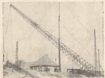
Aerial erection made easy! This is how the new masts for the Post Office station at Cullercoats, Northumberland, were put into position. Hardly a job for the amateur, is it?
