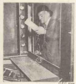
Photoelectric cells foil the smash-and-grab raider by actuating a steel shutter
