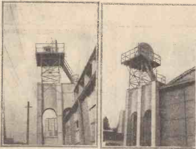
Two interesting views of the aerial system of the 17.5-centimetre aerial assembly erected at Lypmne for testing with St. Inglevert (France)
