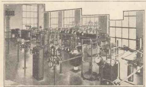
on high power. Part of the transmitting gear of the new Vienna (Bisamberg) broadcaster, which uses some of the biggest water-cooled valves in Europe Vienna on high power.
