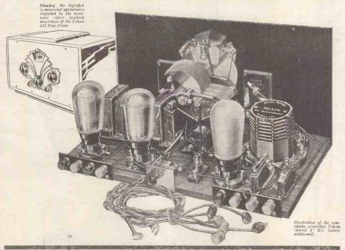
The TELSEN 'ASTRAL 3' embodies every ultra-modern refinement, including slow-motion disc drive control, air-spaced logarithmic condensers, decoupling in circuit, separator control and handsome silver oxidised escutcheon plate.
