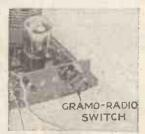
set the radio-gram switch wiring is in the detector circuit and the switch should be kept close to the detector holder, as shown here. The switch is seen mounted at the back of the set on a separate terminal strip near the detector holder
