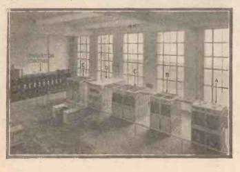
Here are the five panels of the North Regional transmitter. There are two C panels, these carrying the final water-cooled valves. The tuning coils are in the D panel
