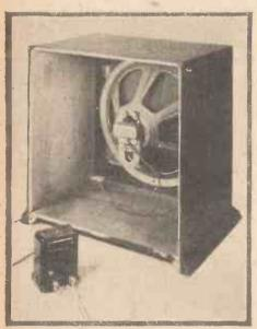
"No speaker can give its best unless insulated from the high-tension current." Here is a speaker fitted with an output transformer
