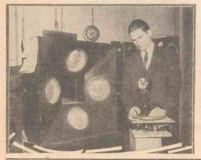
Photo-cells connected to the television transmitter are housed behind this panel with its four windows, and small objects are rotated on turntables before the transmitter so that observers can watch the movement of the image. This is National Broadc a sting Co.
