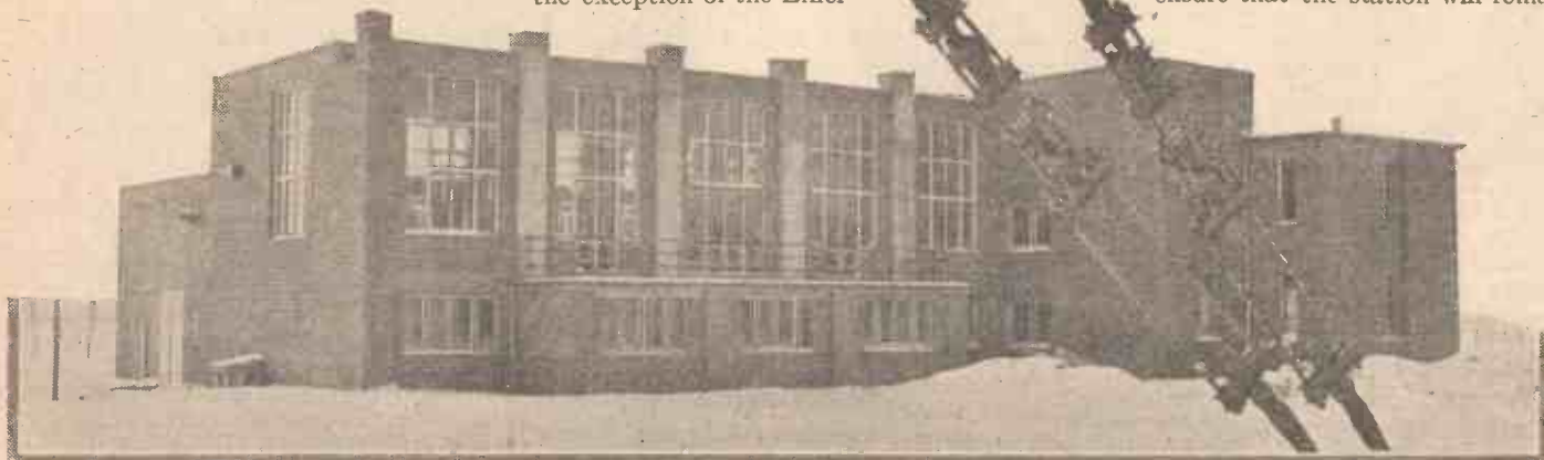
This is the main building of the new huge Warsaw transmitter. The panels of the transmitter itself are in the main hall to the left of the building behind the tall windows, and the machine room is in the right wing. In the foreground are two of the enormous stay adjusters for the 600 ft. high aerial masts
