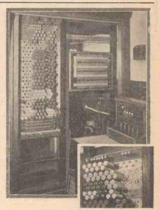
The S.B. Loard relays and fuse panel. Inset is an enlarged view of the relays.
