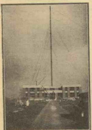
A new glimpse of the rapidly-growing Slathwaite. All three masts are now "up," and the heavy Diesel engines are being fitted. First transmissions are promised by the end of the year
