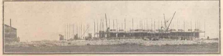
This is the first photograph to be published of the new Northern Regional station at Slaithwaite. The general appearance of the building will be the same as that of Brookmans Park, but the finish will be in red brick instead of Portland stone. As will be seen, the work is already in an advanced stage
