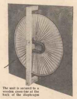
print is to be used, which is the one receiving our strong recommendation, then the Clix socket should be tapped 4B.A. (before the socket is secured to the diaphragm centre of course) and an ordinary loudspeaker cone chuck will then screw firmly into it. The fixing of the button and chuck to the centre of the diaphragm should be done very thoroughly and the diaphragm should be put aside until the glue is quite dry.
