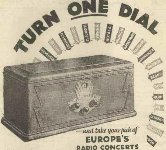
Only three controls on the 1930 Cossor Melody Maker — one for suning, one for volume and one for wavelengths—no coils to change.
