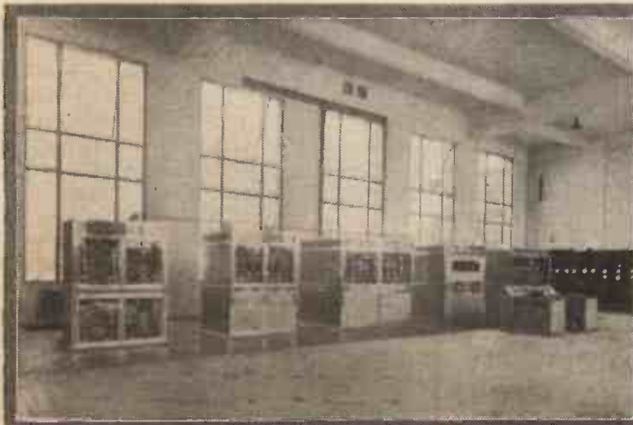
Left: One transmitter with part of main switchboard. Right: The 12,000-volt D.C. generators
