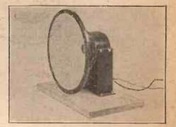
Rotor moving-coil loud-speaker of novel design
