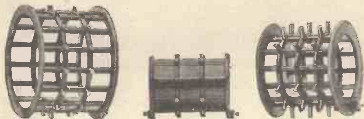
Fig. W 23.—The Coil Formers.
