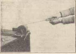
Covered wire, like Glazite, can be straightened and tiffened by nipping a bared end in a vice and stretching it by pulling at the other bared end with pliers.
