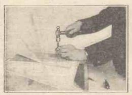
"A.W." blueprints can be used as panel drilling templates. Place the blueprint square on the panel and centre-punch the holes indicated.
