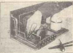
When testing the receiver, insert the valves by holding the anode pin with the first finger to avoid a burn-out.
