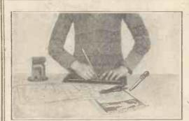
A gramophone needle in the end of a wooden rod makes a simple scriber for marking out an ebonite pavel from blueprint instructions.
