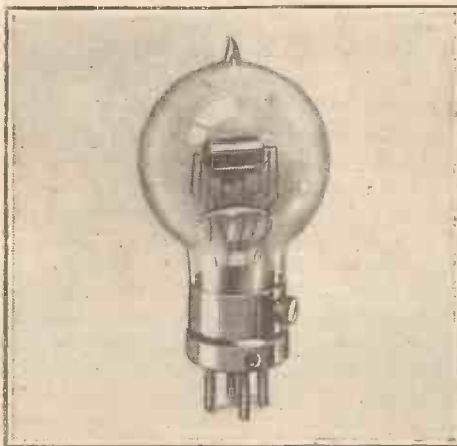
The Tetrode Four-electrode Valve.
