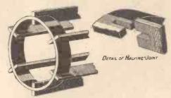
Construction of Low-loss Coil Former.
