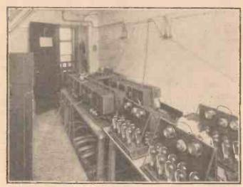
Amplifier control room with Marconiphone power and control amplifiers.
