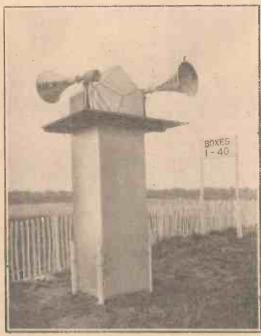
One of the many pylons used for Marconiphone loud-speaking apparatus.
