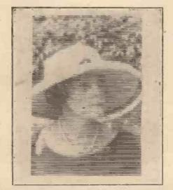
Fig. 4.—Enlargement showing Composition of Telegraphed Picture.
