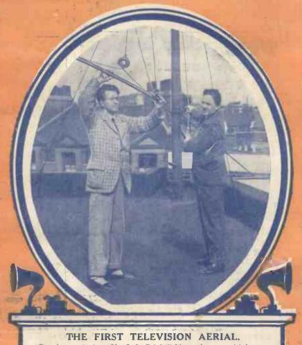
The photograph shows Mr. J. L. Baird (left) erecting an aerial for use with his system of wireless television.
