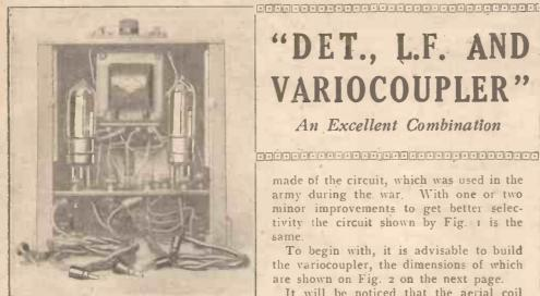
Photograph of Rear of Receiver with Back Removed.
