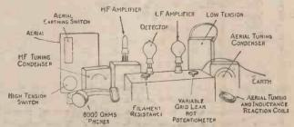
Photograph and Key Diagram of the Three-valve Receiving Set constructed by Mr. J. Seabrook, of the South London Wireless and Scientific Club.
