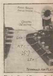
Fig. 4.—Crystal Detector Panel
