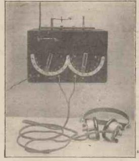
Photograph of Simple Receiving Set made by Mr. F. E. Huson.
