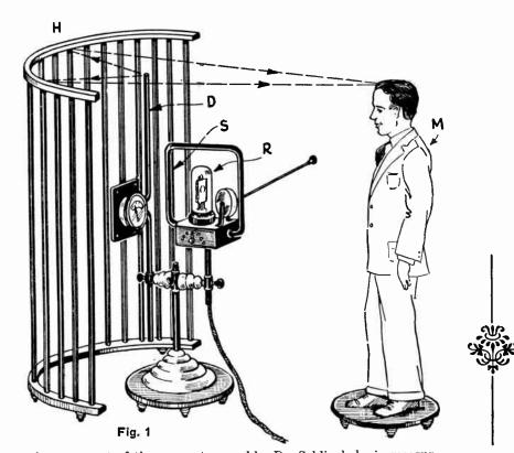
Arrangement of the apparatus used by Dr. Schliephake in measuring and observing the effects of short waves on the human body, absorption, et cetera. H, parabolic reflector formed of wires; D, antenna, charged inductively by the coil S; vacuum tube at R, and beside it wave changing condenser; subject at M.
