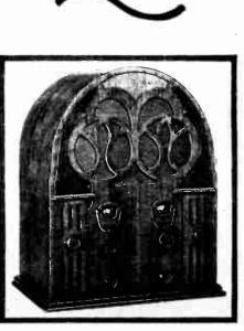
Two-dial "dual" receiver, tunes from 20 to 600 meters; without "plug-in" coils.
