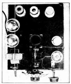
Top view of the 5-meter superheterodyne.
