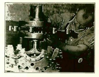
Fig. 154. Assembly of crankshaft and connecting rods in rear half of crankcase and Guiberson radial Diesel engine.
