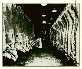
Fig. 20. Photograph of one section of a large meat chilling and storage room which is kept at very low temperature by means of mechanical refrigeration. Courtesy Carrier Corporation.
