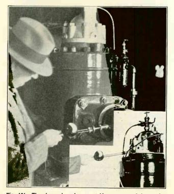
Fig. 104. The above view shows portable pyrometers being used to check exhaust gas and cylinder head temperatures of Diesel engines. (Courtesy Illinois Testing Laboratories.)
