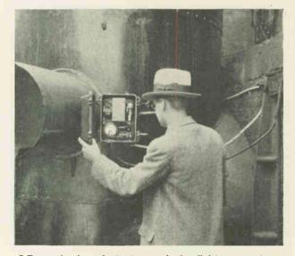
G-E protoelectric smoke-density recorder installed in a power house. It indicates the amount of smoke leaving the chimney.
