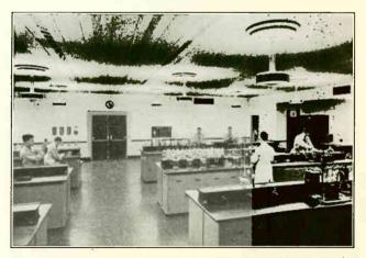
y. 159. Interior view of spotlessly clean air-conditioned chemical laboratory, in the building shown in Fig. 158. The advantages of air-conditioning in chemical laboratories, food manufacturing plants, and fine instrument shops are very apparent. Courtesy National Advantation Courtesy National Aluminate Corp.
