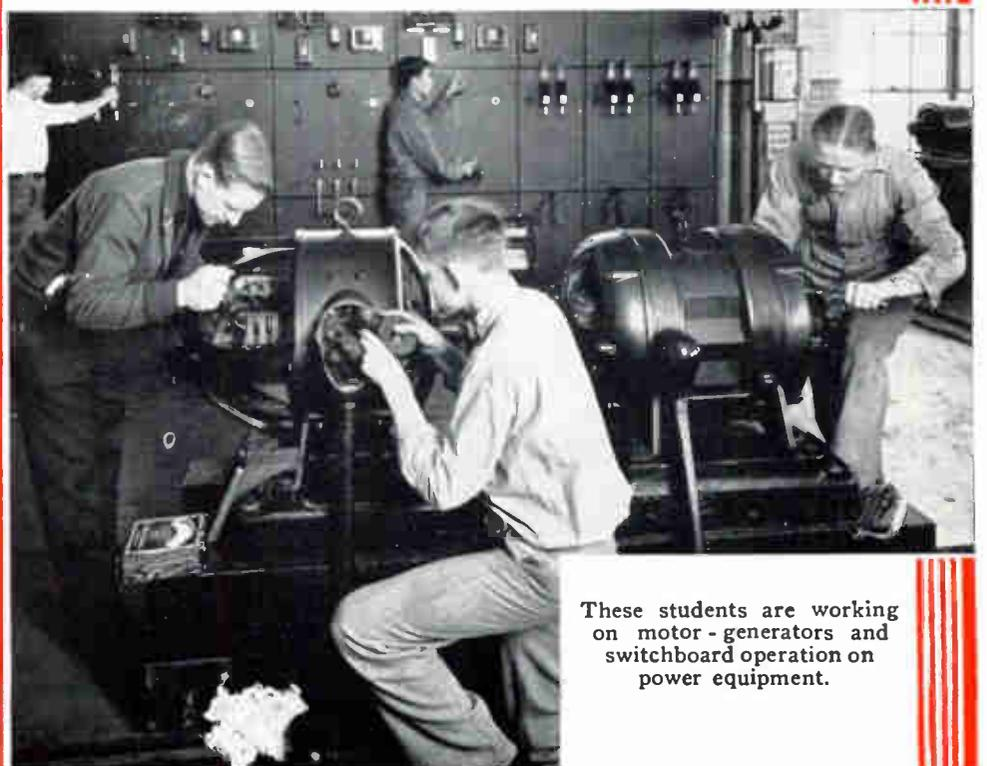
These students are working on motor-generators and switchboard operation on power equipment.
