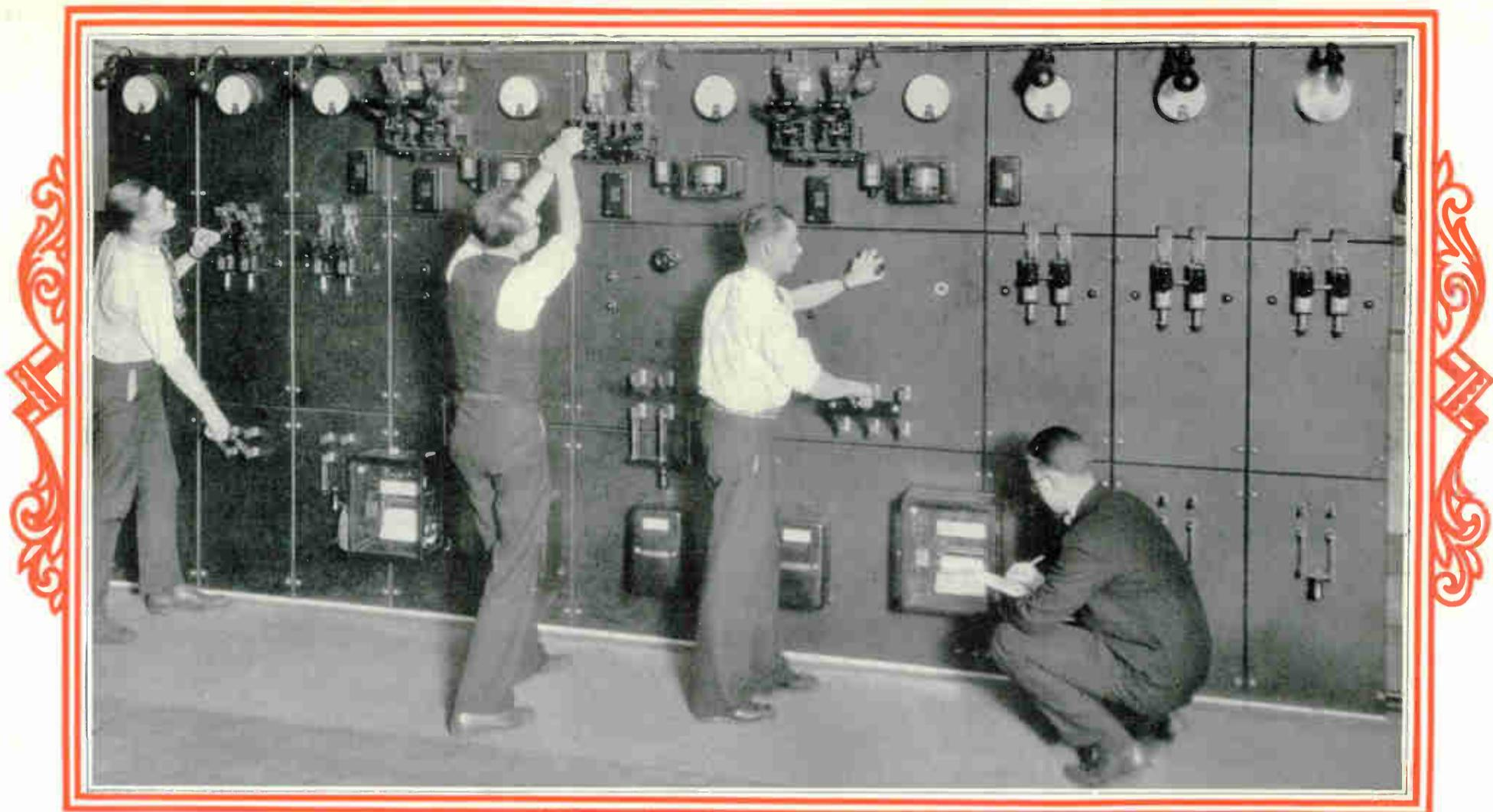
Here are students getting real operating experience on a large power D. C. Switchboard. They are taught to connect and operate generators in parallel, and to take care of circuit breakers, switches and instruments. This kind of training is valuable in power plant or substation operating work, and many of our graduates have good jobs doing this work.
