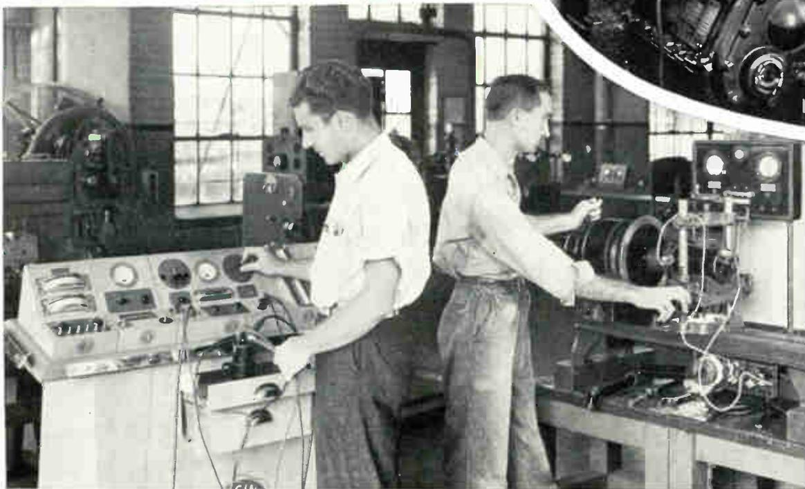
These students are using modern garage type tests units for giving final tests to generators, starters and coils they have overhauled and repaired. This equipment shows you the actual results and voltage of the generators at different speeds, the same as on the car, so you know whether your work is done right. Work on such equipment qualifies our graduates for jobs where services of trained practical men are required.
