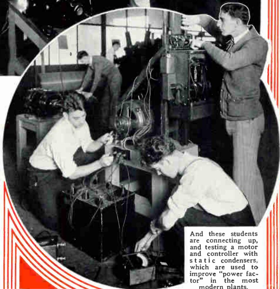
And these students are connecting up, and testing a motor and controller with static condensers, which are used to improve "power factor" in the most modern plants.
