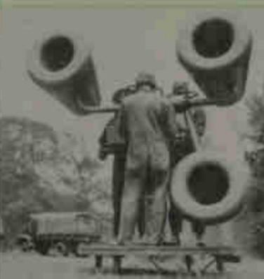
Electronic systems for the Army. (Left) Sound system, known as electronic ear, was of Westinghouse design. (U. S. Signal Corps.)
