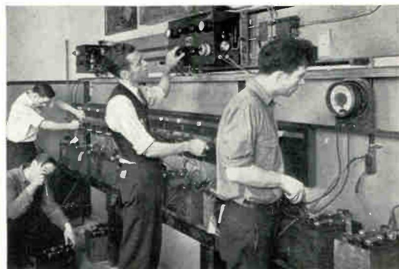
Here they are operating the charging line and equipment of the Tungar type. Both the half wave and later type full wave charges are used here. And you see these students testing the acid, and the voltage to determine the exact condition of the batteries being charged.
