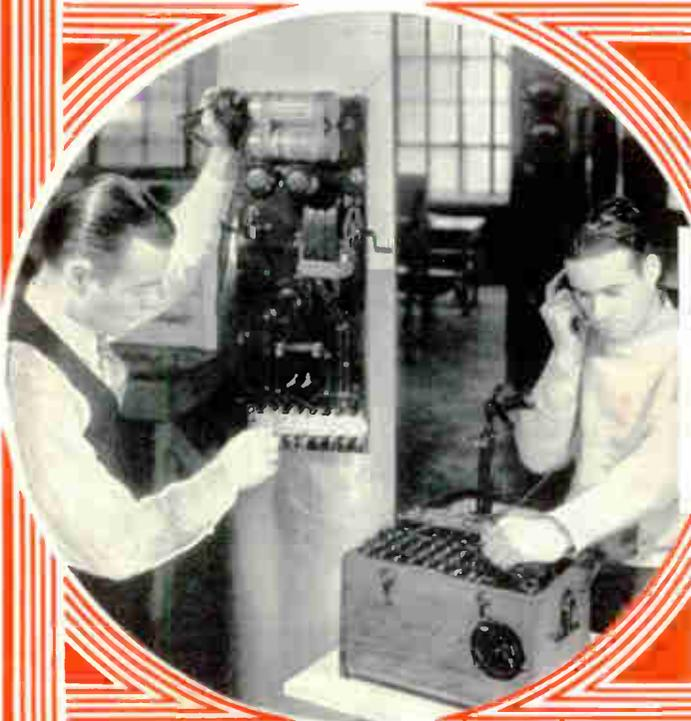
These men on the left are wiring and testing telephones. The instructor explains the operation of each part and then the students wire up the phones and test out their work by talking over them.
