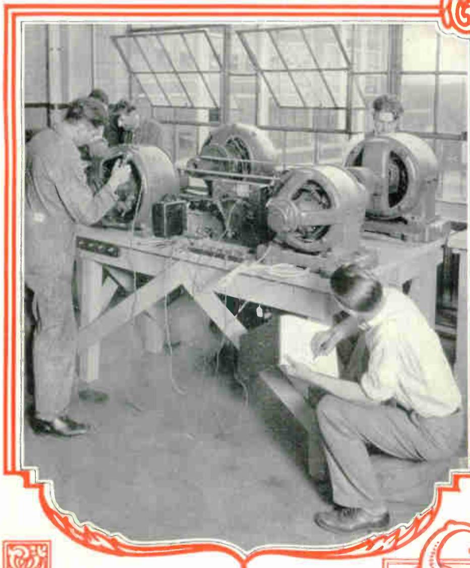
These students are operating and testing motor generator sets, building up voltage, and measuring the output of these units.
