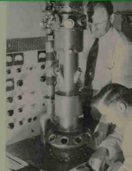
Electronics in Microscopy. The conventional RCA electron microscope, which shows detail up to one-hundred-millionth of an inch, 100 times as fine as that of a good optical microscope. Unprecedented discoveries in bacteriology, chemistry, mineralogy and other fields are practiced with its aid.
