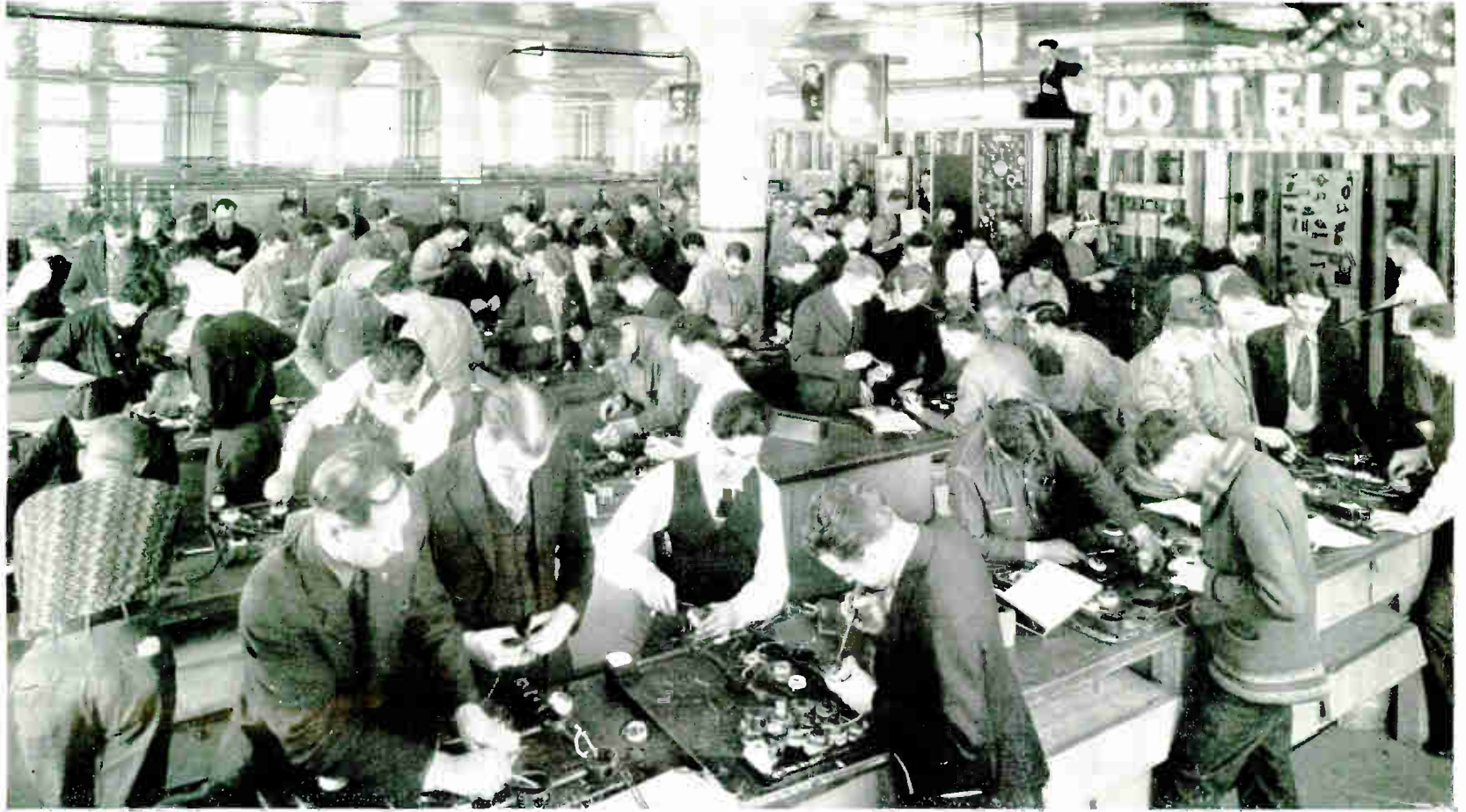
General view of a section of the electrical wiring department. Notice the large and well lighted shop. The men are wiring and testing light control circuits in their first small conduit layout, and getting real practical experience in the handling of tools and different kinds of switches.
