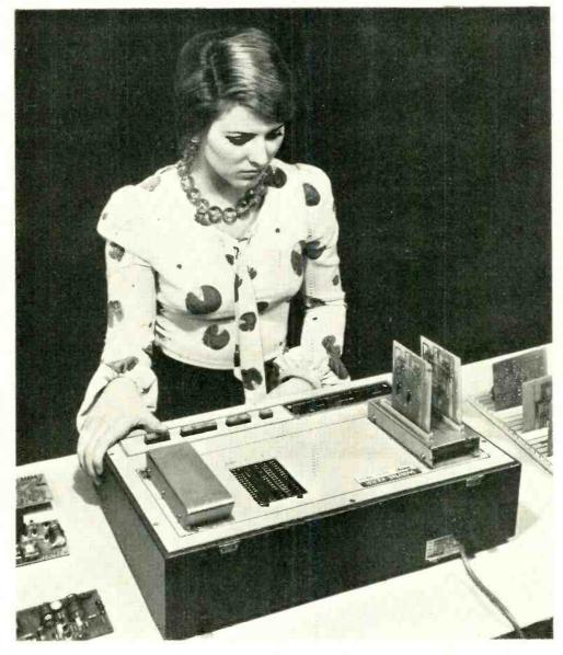
Easy to set up and operate, the Swift Digital A.T.E. checks digital printed boards containing T.T.L. circuits or T.T.L. compatible functions.
