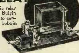
A special electro-magnetic relay utilising the well-known Bulgin efficient-magnet system, to conserve the flux. With a bobbin resistance of 7,000 to 7,500 Ω D.C., it is wound with enamelled copper wire, well insulated. The adjustable secondary contacts form an S. P. D. T. switch. Handing capacity 1-A at 2-volts to 10-mA at 250-Volts.
