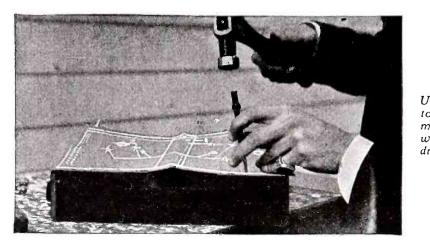
drill the various holes as indicated. The platform is now ready for the subsequent mounting of parts and for wiring. A coat of shellac or varnish, at this time, provides an attractive finish and also serves as a protection against moisture.
