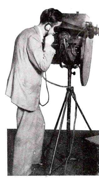
The television cameraman at work, focusing his picture by means of the "monitor" view-finder, while checking on his signals by means of head-phones.
