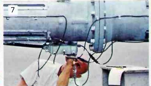
(7) Connecting the de-icer into the junction box on a TFU-45J UHF Pylon antenna. This is one of a new family of moderately priced UHF Pylons.
