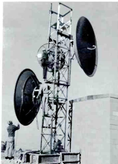
Waveguide plumbing goes on a 10 foot dish at the Little Belt site near Lewistown, Montana. Despite the rugged appearance of the installation (and it is!) wind later tore the dish from the mounting tower and sailed it 200 yards through the air doing \$1500 damage.
