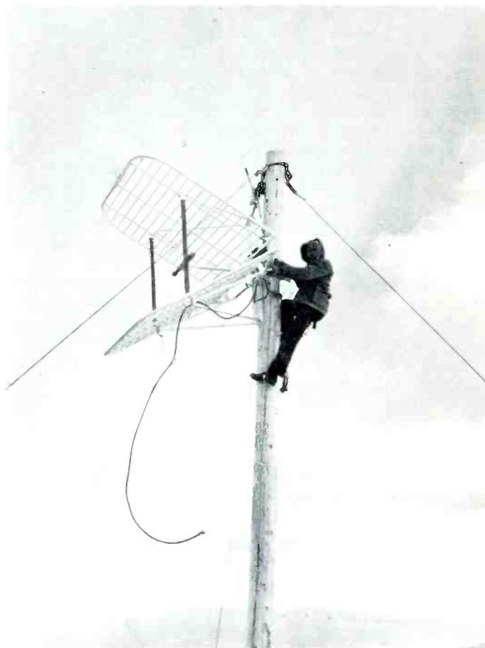
Jampro Antenna Products Corner Reflector installed at Clinton, B.C. contains de-icer element to keep the ice from coating over the array. The antenna, an important investment with any translator, cost nearly twice as much as the translator itself, but is considered worthwhile in view of the particularly bad weather conditions it will experience. Four to six months per year, the antenna and site will be inaccessible.
