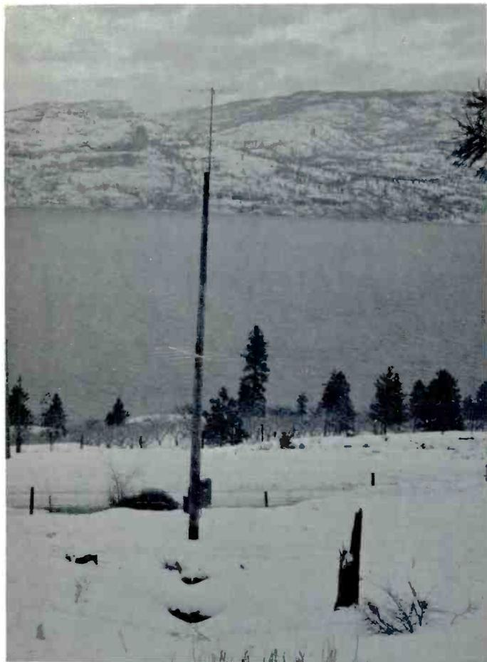
Pechlond, B.C. T-5 translator installation consists of a telephone pole, and two yagi antennas—one for receiving, one for re-broadcasting. In a land where trees outnumber people 10,000 to 1, every microvolt of signal counts here!
