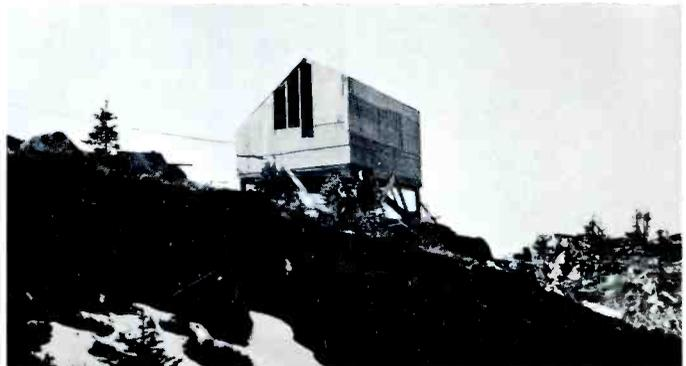
A trick borrowed from Idaho CATV systems, this shed houses receiving antennas on Botani Mountain near Lytton, B.C. at the 7,000 foot level. One side of the housing is fibreglass to let the R.F. in, and keep the snow and weather out. Snow frequently covers the shed with 14-20 feet on level areas during a heavy winter.
