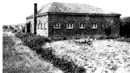
Apparently a farm building of red brick with green shingled roof and with windows suggesting innocent domestic purpose. Actually, a Nazi "fortress" with walls and roof of reinforced concrete, four feet thick.
