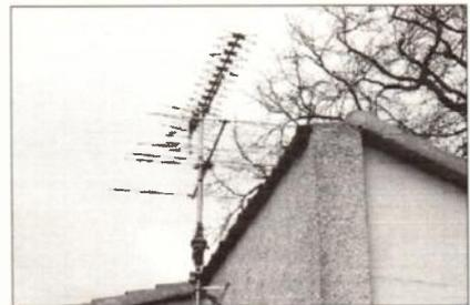
George Garden's DXing installation comprising an XG14-type u.h.f. array with a 4-element f.m. array below.
