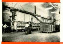
The largest sheets of mica ceramic insulation available (19% x 29%) made only by Electronic Mechanics, are produced in this firing kiln followed by 12 to 36 hour anneoling in the Lehr. This removes all internal stresses and strains in the sheets assuring great physical stability.
