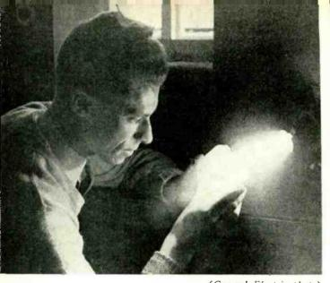
(General Electric photo) Detecting flaws in quartz by Klieg light
