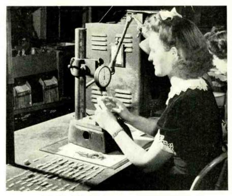
Sorting blanks into thickness groups preparatory to lapping (RCA-Victor photo)
