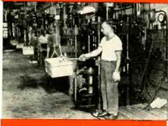
One of several batteries of precision presses for injection and compression malding Mykroy. Here ore produced a large percentage of all molded mico ceromic ports required for the wor effort.
