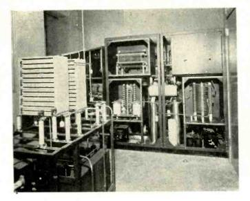
Behind the scenes at Nashville's 50-kw radio station WLAC. This view shows details of the Western Electric condenser and switch assembly and of the tank circuit components.
