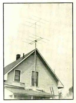
The double W6QLZ beam which was in use from July 20 to September 24, 1941, by W8JLQ, Toledo, Ohio. The stacked affair has since then been replaced by a single section of the array.
