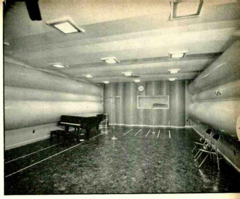
The latest thing in b.c. station studio construction: WFAA-KGKO, Dallas. The arrangement of cylindrical wall surfaces and sound-absorbent material is for acoustical purposes. Photo courtesy Armstrong Cork Co.
