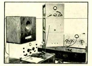
The station at W6OUE. On the left is the RME-69 and its speaker, then the 160meter 'phone rig and the 40-meter c.w. r.f. section. In front of the receiver is the Braille guide and punch.
