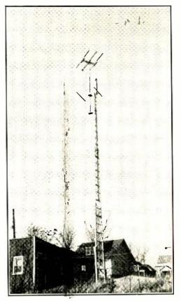
The 56-Mc. horizontal and vertical 56-Mc. antennas in use at W9QCY.
