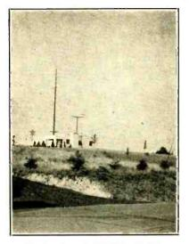
The location of W8CIR. A 3/2wave vertical is located atop the telephone pole and a 7-element Yagi mounts on the rotary affair on the roof.
