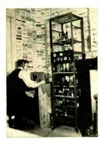
ON4HC, owned by S. Van de Wouwer, near Antwerp, Belgium. The rig uses a pair of 10's in the final amplifier with 50 watts input.
