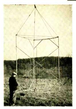
Figure 4. The 56-Mc antenna with squarecorner reflector at W8JK. The half-wave radiator has been retouched to show its position more clearly. The transmitter is at the lower end of the half wave. The power supply is on the box under the reflector. The sides of the reflector curtain are substantially flat and meet at a right angle although due to an illusion it appears in the photograph that the reflector is slightly curved.
