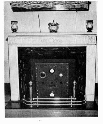
• Add, unusual transmitter locations, that of W8BXN. The rig is a 150-watt allband affair remotely controlled from the living room desk, and was installed in the fireplace simply because there was no suitable space elsewhere.
