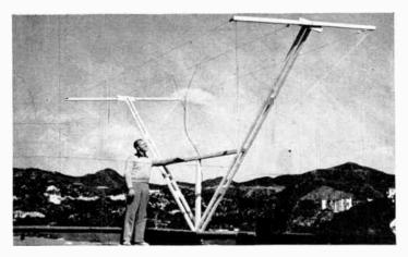
FIGURE 1. The original wire-and-insulator three-element beam installation at W6PKK. The OM himself bracing the supporting structure.
