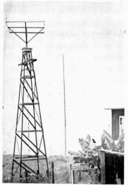
FIGURE 5. The rotary in use at K60QM. The three elements of the array are rather indistinct but they may just be seen mounted upon the rotary structure atop the tower.
