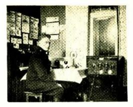
LA4K, Lorenskog, Norway. The transmitter uses an RK-20A in the final with 100 watts input on c.w. Operator is a policeman and 34 years of age.
