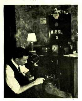
W1BRL the station of Wink Wight, taken by the OM. 27 watts input, crystal controlled, fone and c.w. on 56.096 Mc. The receiver is a resistance-coupled superhet.
