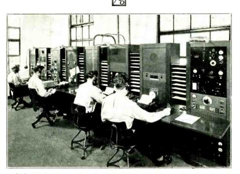
E.A.L. ground station at Miami, Fla. Transmitters are remotely controlled. The unit to the extreme right in photograph is the frequency standard used for periodic checks upon the equipment.
