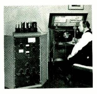
The complete transmitter mounted in an enclosed relay rack.
