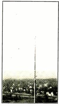
The Wheaton. Illinois, Police transmitter uses this concentric-line-fed "J" type antenna. It is mounted atop a water tower, high above the closest traffic, and used both for transmitting and receiving.
