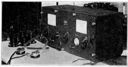
Marshall Short-Wave Receiver, as Used by Navy
