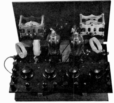
Short-Wave R.F. Amplifier with Screen-Grid Tubes
