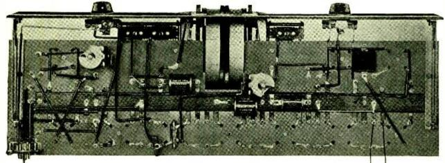
Bottom View, With Capacity Connector Strip in Place. RADIO FOR OCTOBER, 1927
