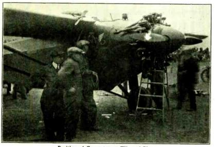
Position of Generator on Wing of Plane. RADIO FOR OCTOBER, 1927
